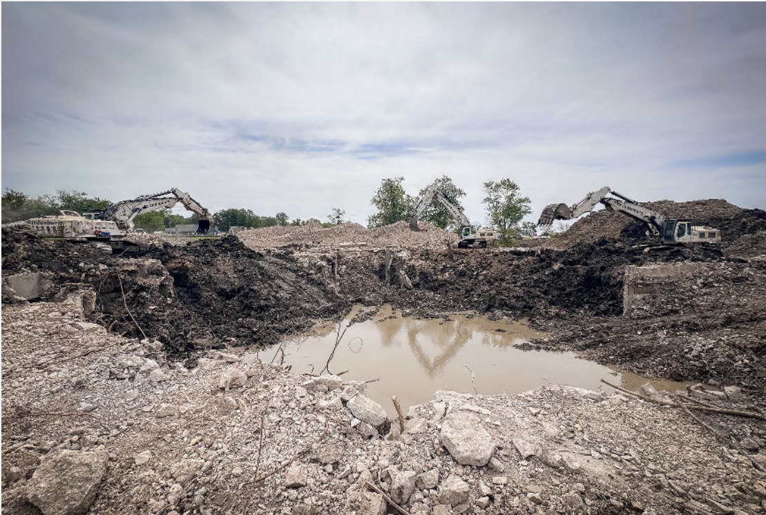
Basement excavation at Spruce Hall
