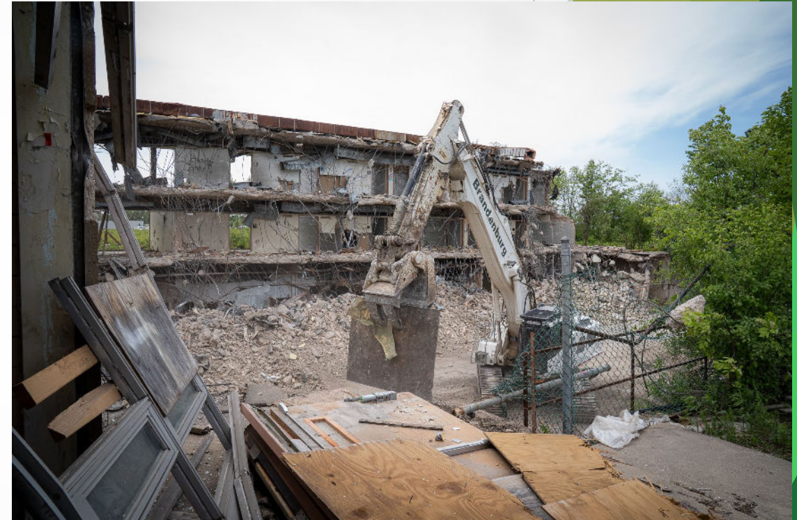
Demolition and debris removal at Oak Hall
