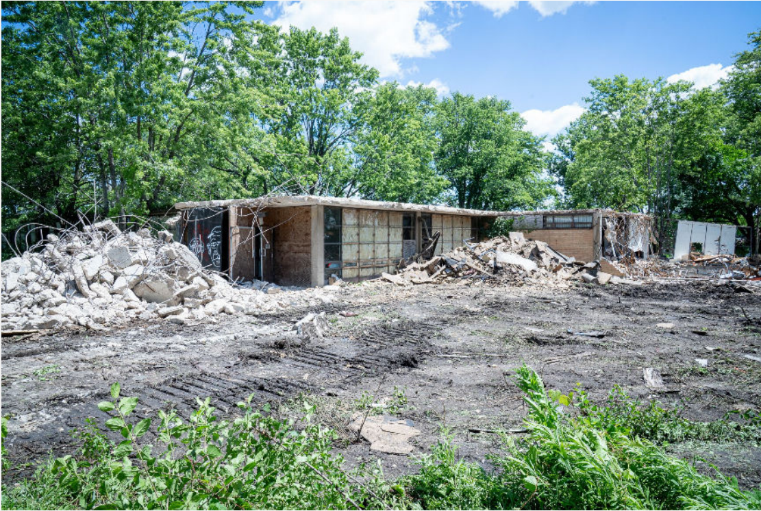
Demolition at Willow Hall
