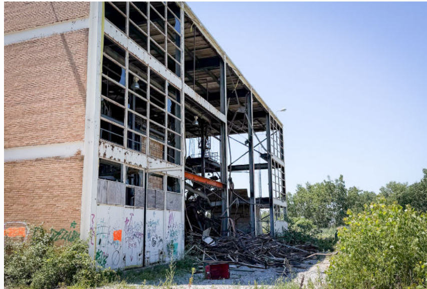
North side of the Powerhouse
