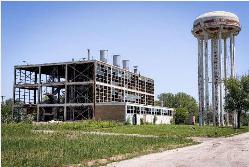
Demolition work at the Powerhouse
